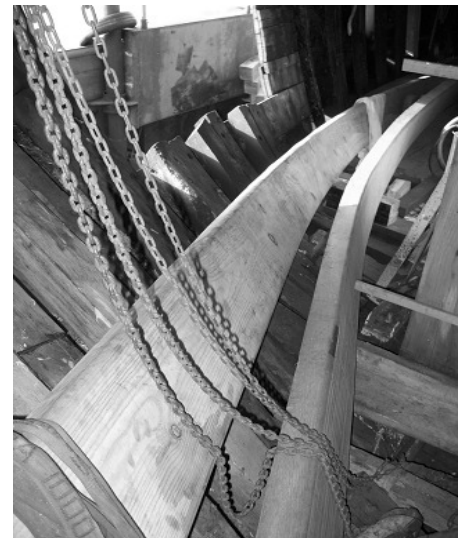
Timbers inside Pudge waiting to put in place
